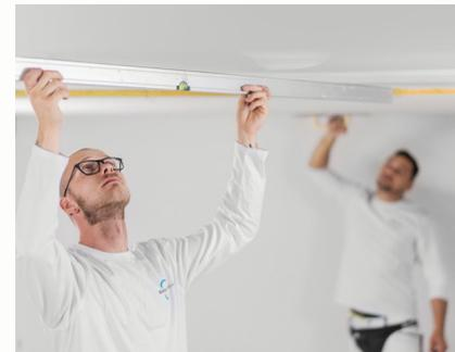
**2. Adhering the acoustic panels** The acoustic panels are easily applied to the substrate with an adhesive. For curved surfaces the panels are cut and prepared accordingly on site.
