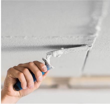
**3. Filling the joints** Joints are expertly filled and then sanded so that they are not visible in the final state.
