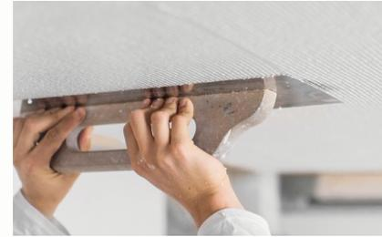
**5. Application of the base coat** Apply, smooth, dry — in these simple steps experienced installers install the perfect base coat. In single-layer systems, this also corresponds to the final layer.
